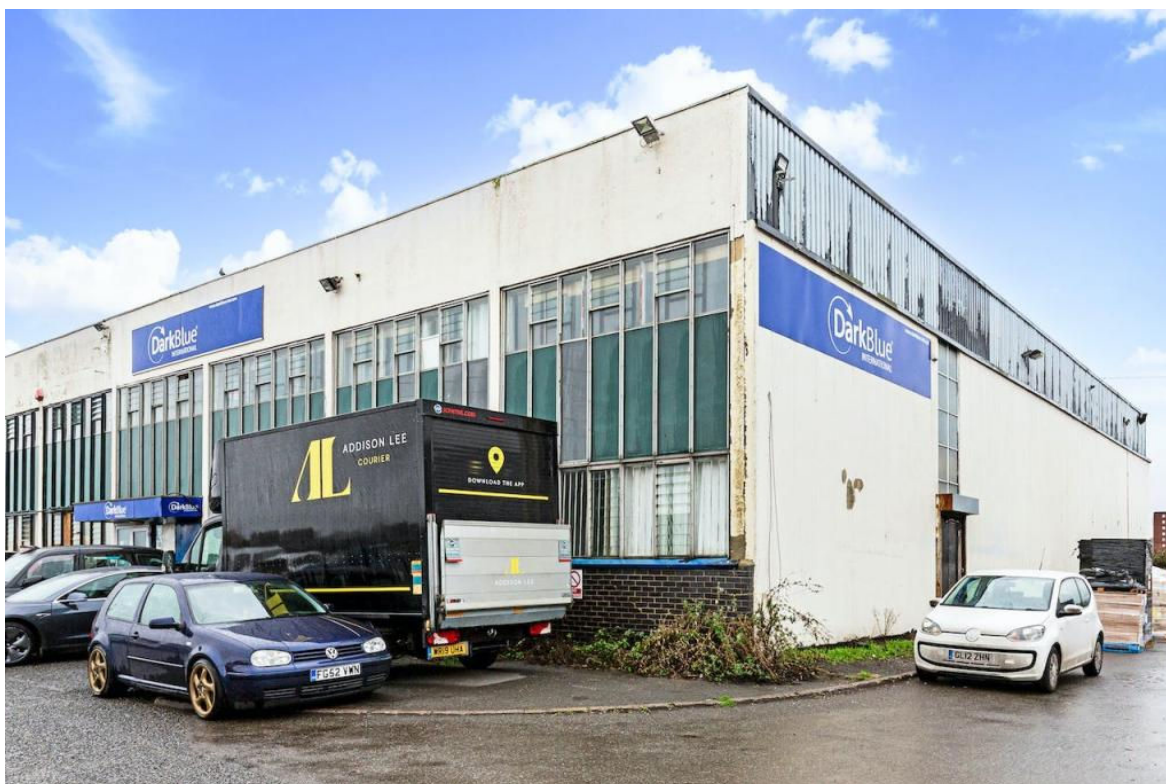
Figure 2: External view of building
