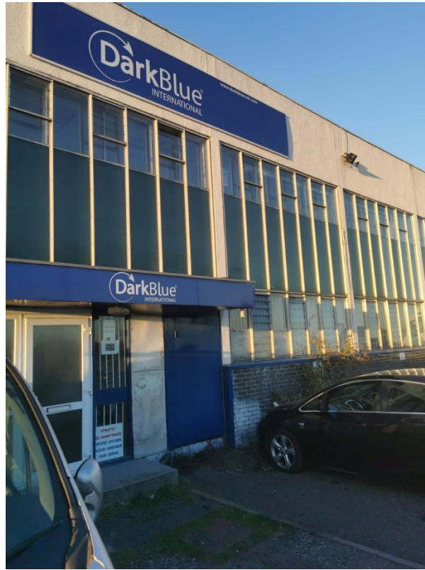
Image 3 - Current Frontage of LDN Riverside Unit
